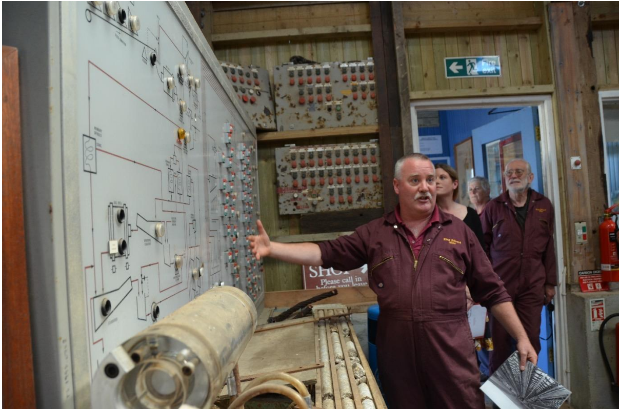
Figure 13: Nigel speaks of the mill control panel
