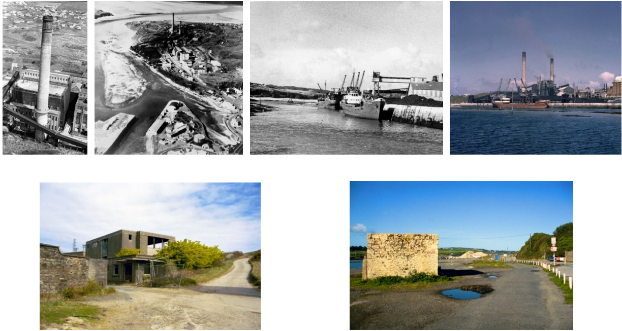
Figure 27: The power station and many other industries used to be based on North Quay. Archive photographs by Hayle Community Archive and derelict images by Dr. Simon Clarke.
