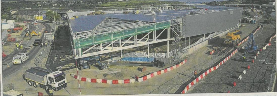
The new Asda supermarket development on South Quay, Hayle.
