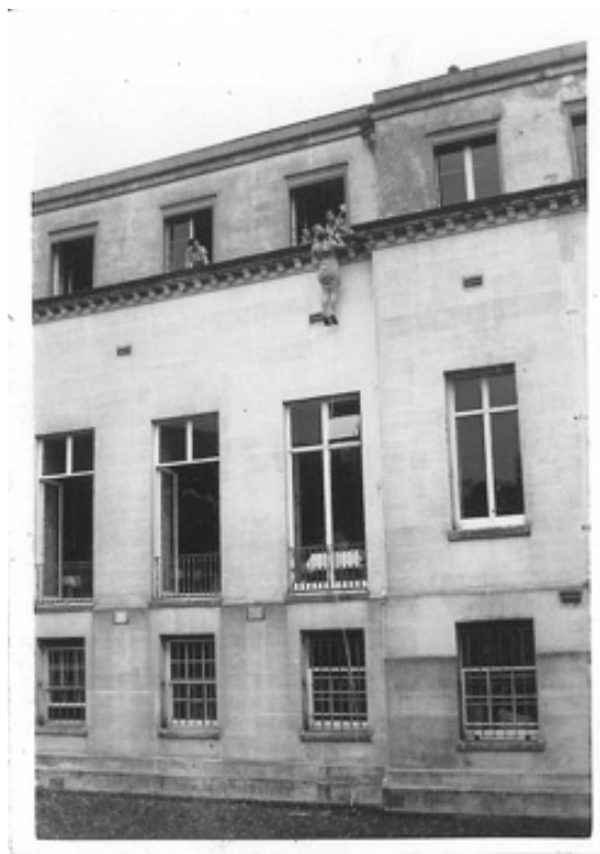
Figure 37: Stratton Park, n.d. , The Baring Archive
