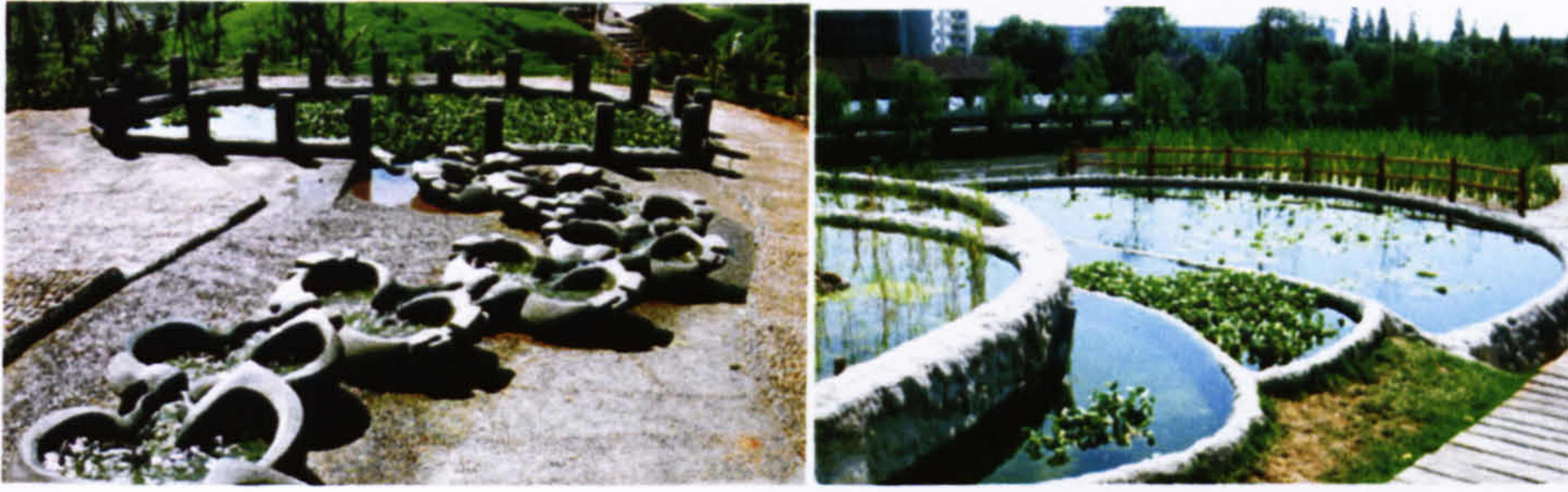
10. aeration system, bio flow forms wetland ponds with water-purifying plants
