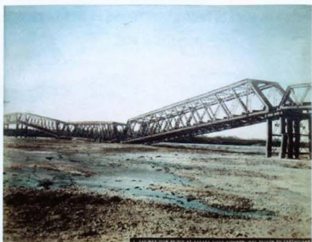
**Fig. 1.7** Railway Iron Bridge at Nagara River Aichiken, was broken by earthquake
