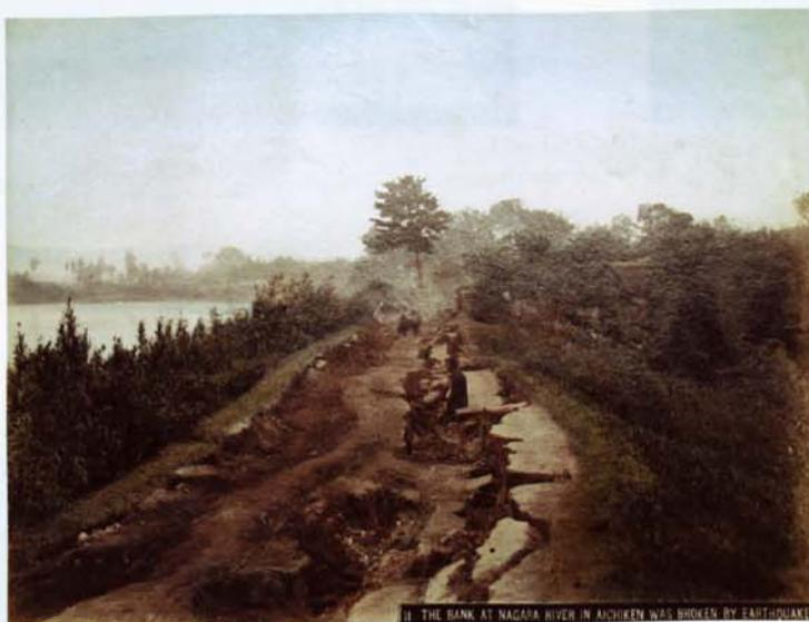
**Fig. 1.10 The Bank at Nagara River in Aichiken, was broken by earthquake**
