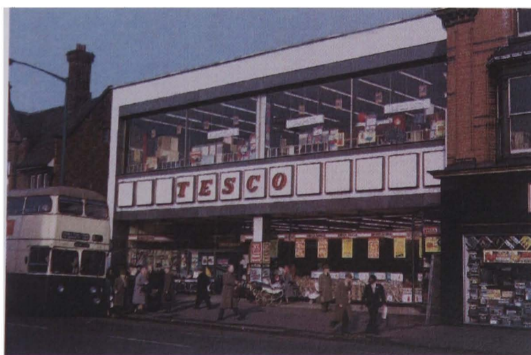
Picture 6 Tesco Birmingham showing canopy (Tesco archive)
