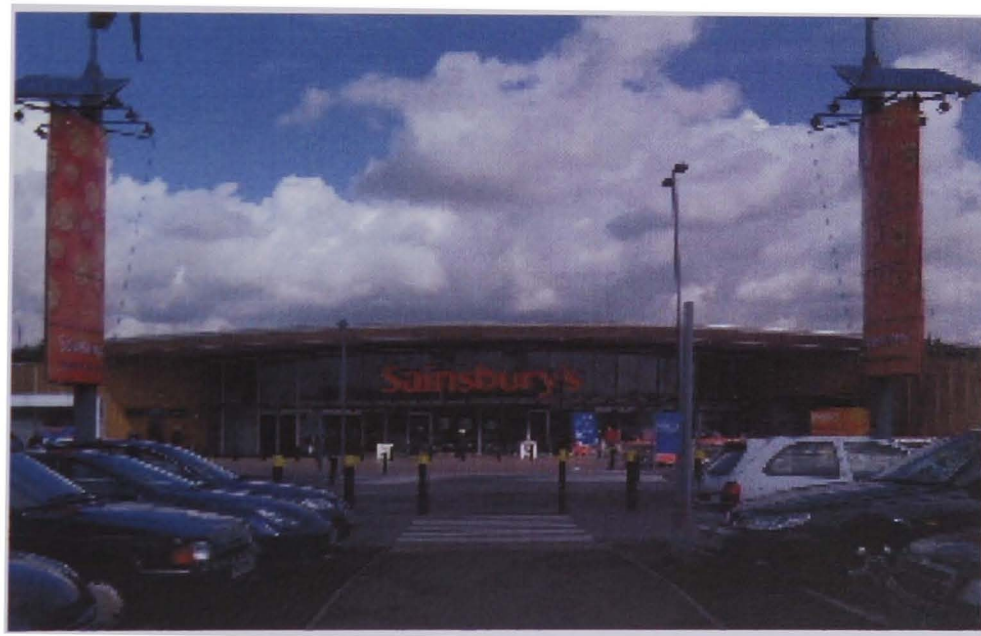
Picture 54 Sainsburys Greenwich-showing the front of the store with masts (Kirby)
