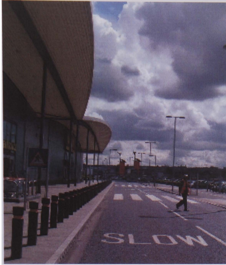
Picture 56 Sainsburys Greenwich –view of the store 2004 (Kirby)
