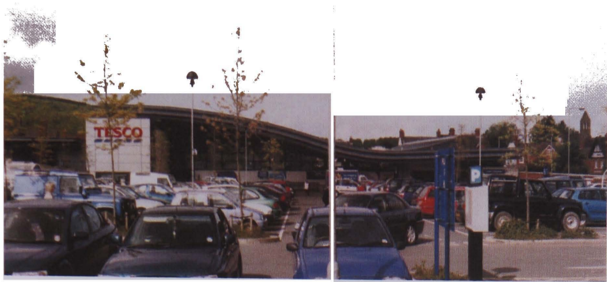
Picture 46 Tesco Ludlow -The store from the car park showing the curving roof (Kirby)
