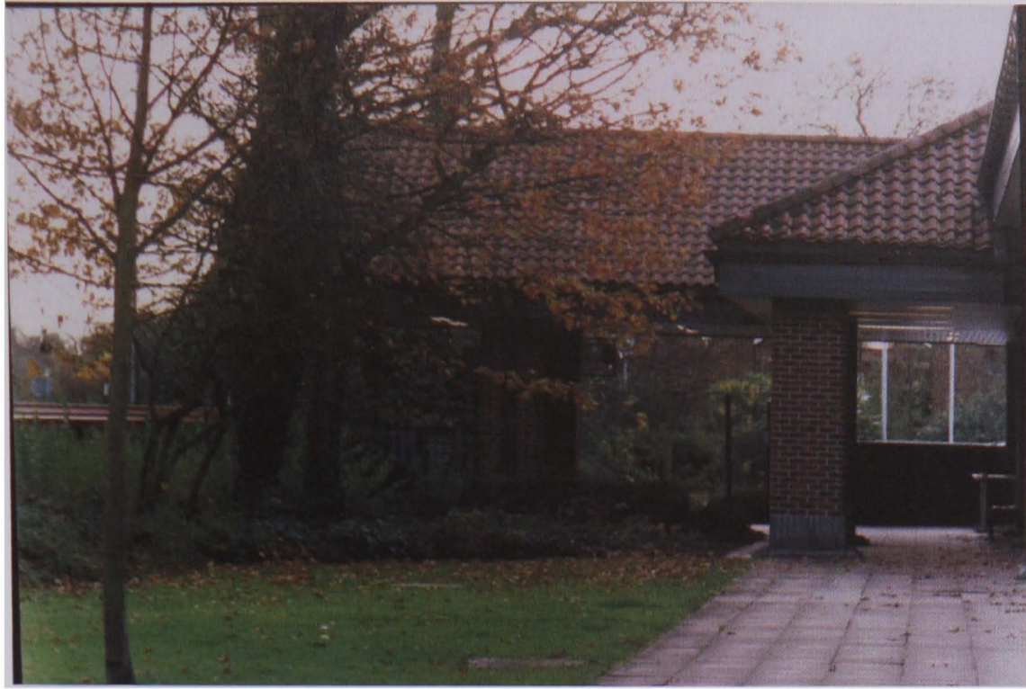
Picture 39 Side view of the pedestrian entrance Winchmore Hill (Kirby)
