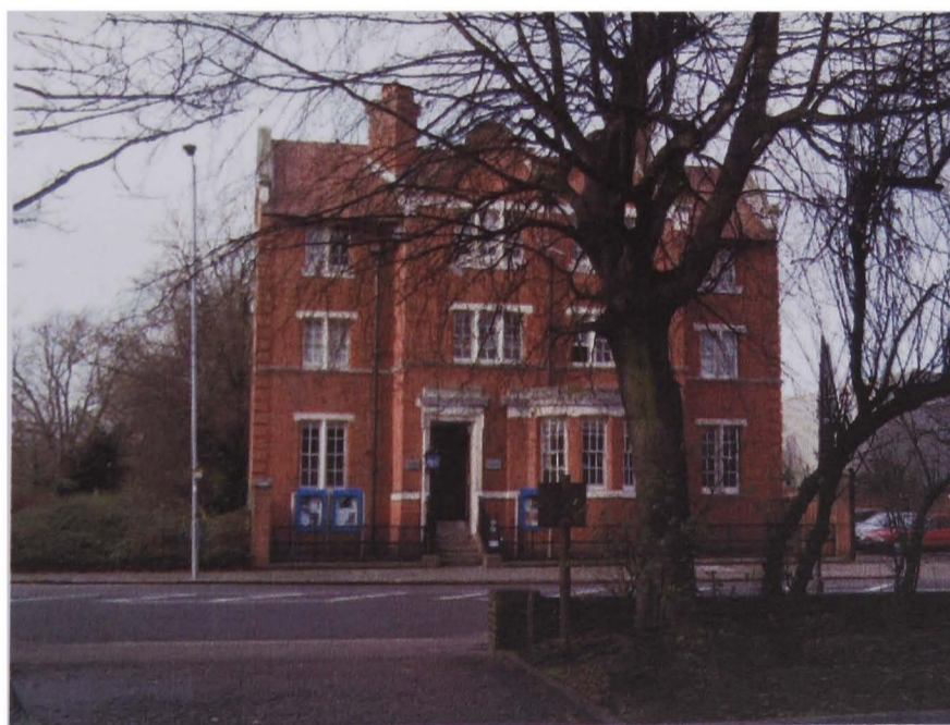
Picture 35 The Police Station Winchmore Hill (Kirby)
