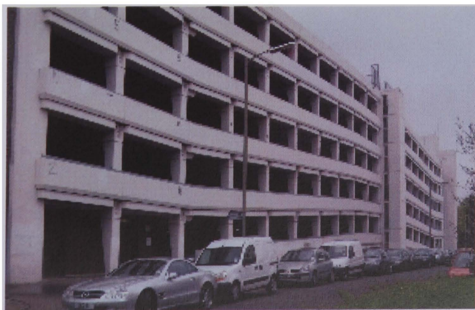
Picture 66 Orpington –the multi storey car park
