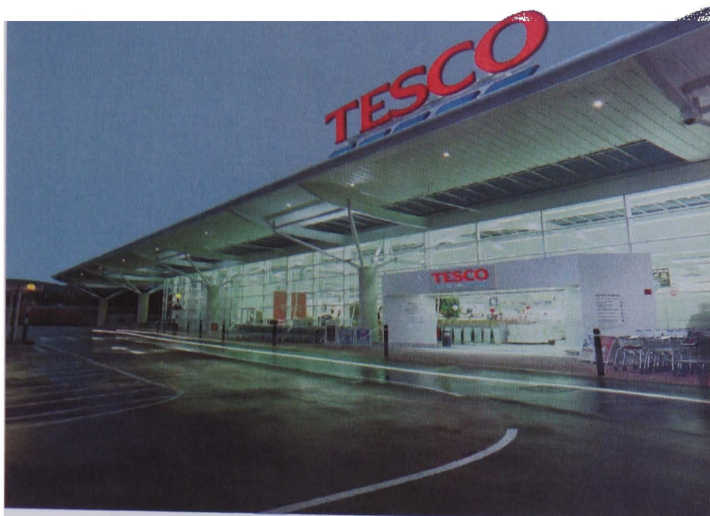
Picture 30 Tesco Sheffield showing exposed ceiling and air barrier (Tesco archive)
