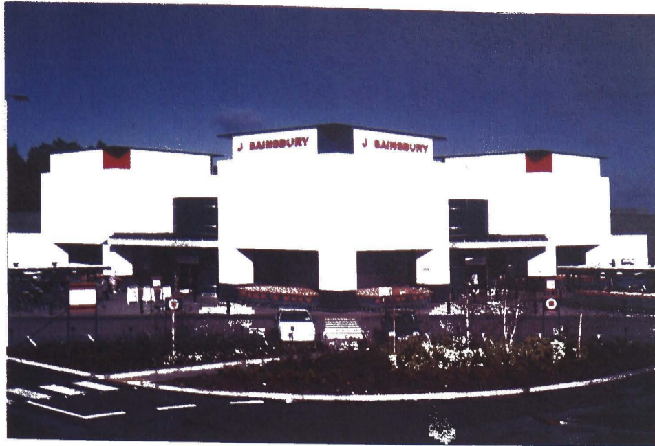
Picture 27 Sainsburys Harlow (Sainsburys archive)
