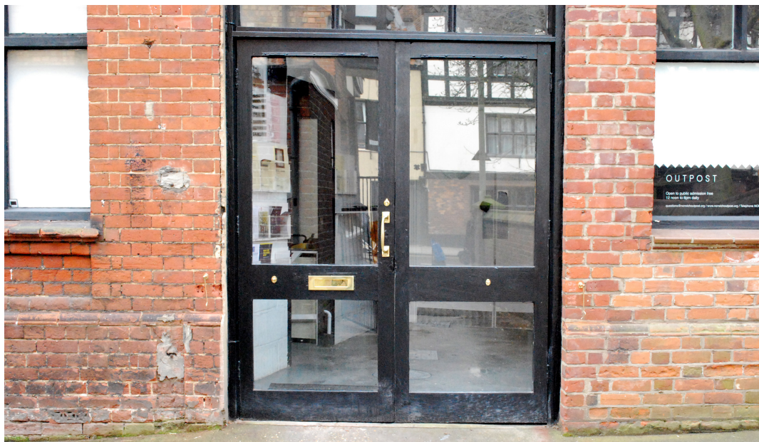
Gallery doors before and after renovations (Research images) 2010
