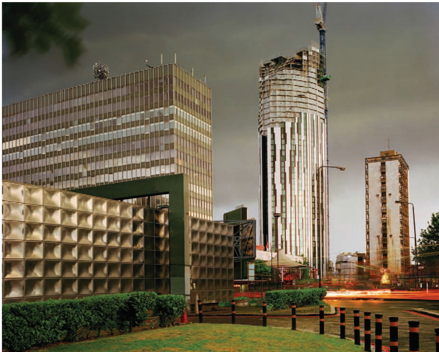
“A real sign of the coming regeneration of the Elephant and Castle” and “the next London icon” said Simon Milton, Deputy Mayor of London, watching the topping out of the Strata tower, a new 43 storey residential block, that will “truly put the Elephant on the map of London”. The adjacent Draper Tower, now dwarfed by the Strata, was once the tallest block of flats in London and home to City workers, who enjoyed magnificent views over the Capital. Most of the available apartments in the Strata Tower sold very quickly despite prices up to 2.5 million pounds.
