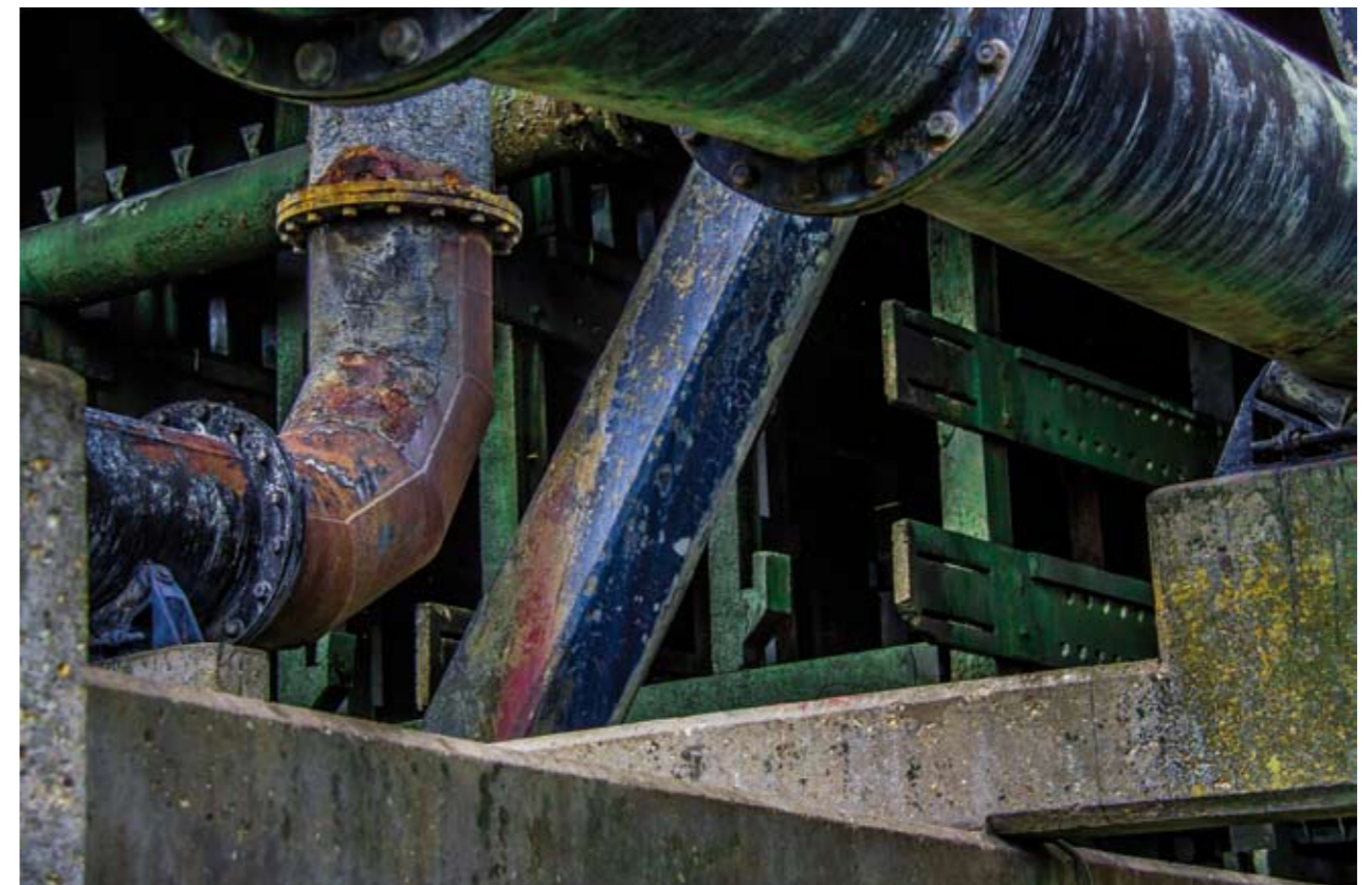
Clockwise from above: "Inside a cooling tower" and "Pillars at the base of a cooling tower", Mick Furby, "Pipes going into a cooling tower", Bob Brown
