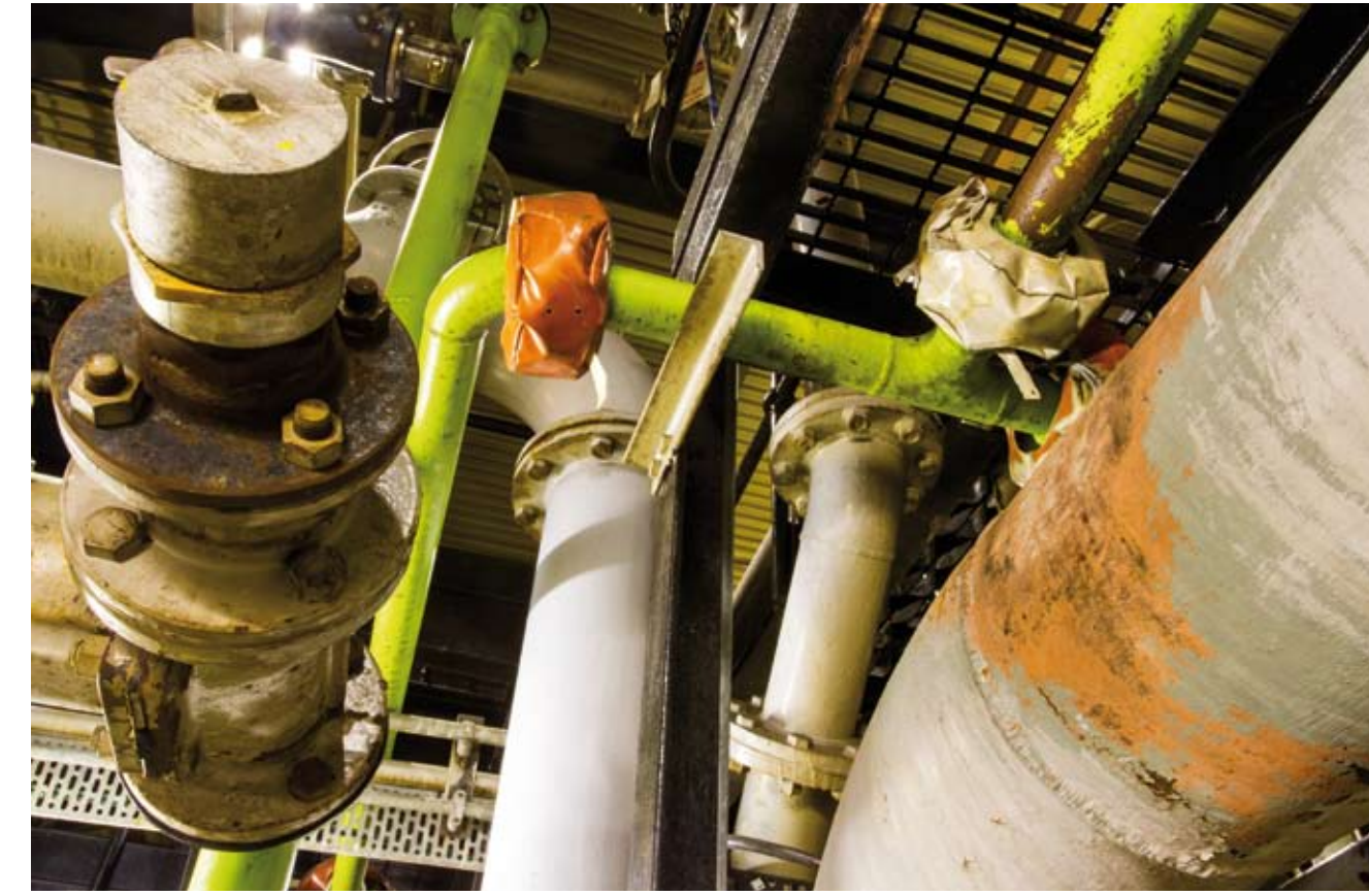
Clockwise from top left: "View of water treatment plant 1", David Belcher, "Water treatment plant 1 pipework", Mike Foster
