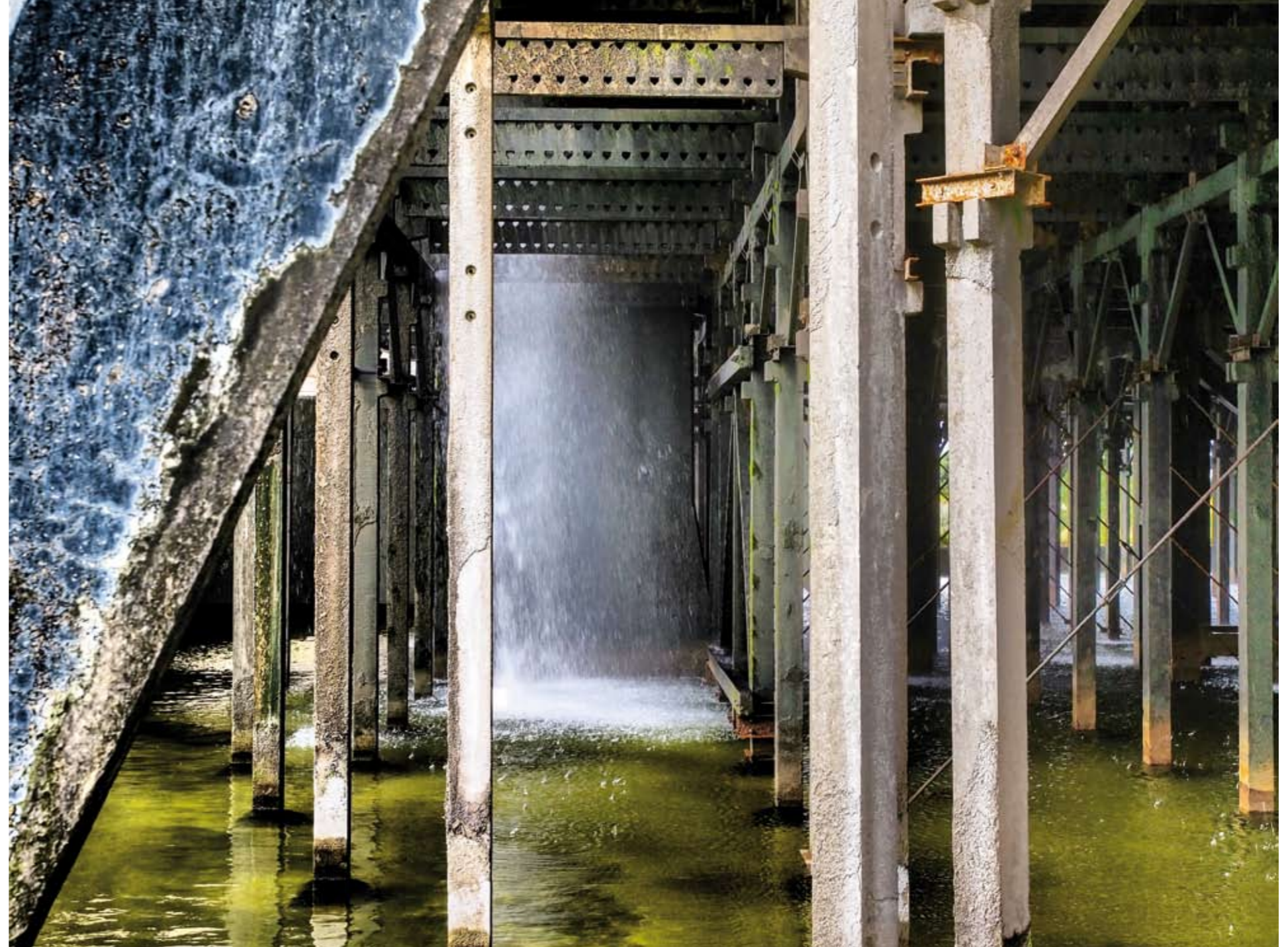
"Underneath a cooling tower", Phil Childs
