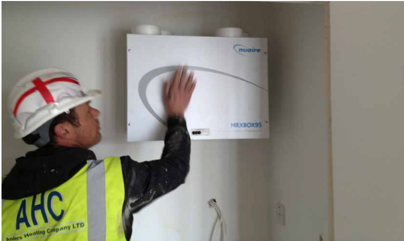
Installation of Nuaire's ventilation product
