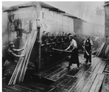
Fig. 4: Steaming ovens at the Thonet factory in Bistritz c. 1920 (Vege sack, 1996: 70)
