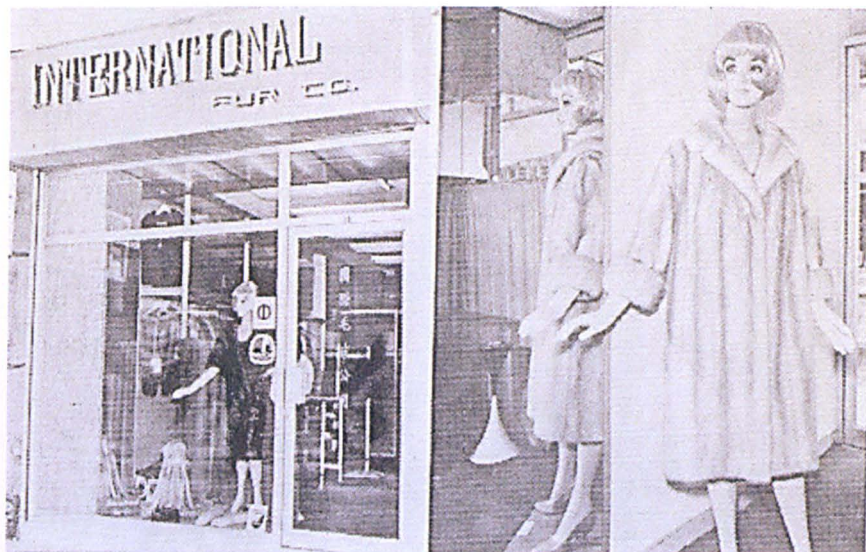
Figure 60 International Fur Company store exterior 1970
