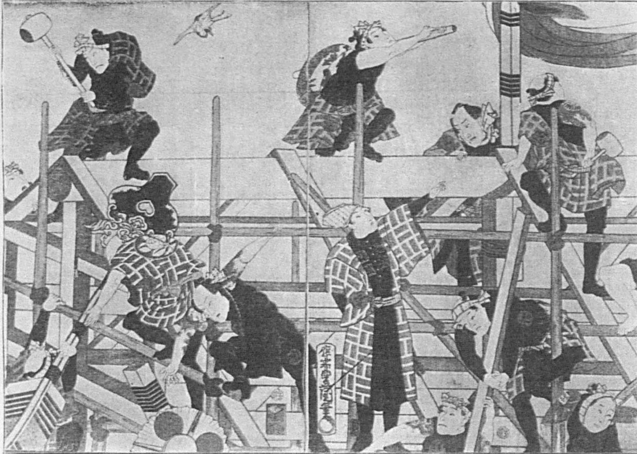
ERECTION OF A HOUSE: REPRESENTED BY ACTORS.
