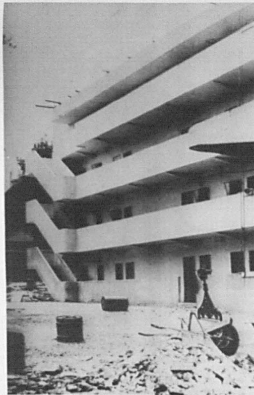
39 (51) Work in progress at Lawn Road.
