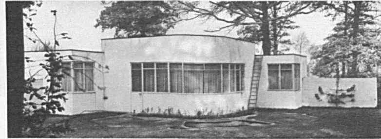
ONE-STOREY HOUSE on a site sheltered by trees on the north and open to fine views on the south. A tank room—often a problem in flat-roofed houses—is fitted in at a convenient break in roof level, where the height of living-room increases. The plan is a development of the basic "Sunspan" plan, exhibited at Olympia in April, 1934.
