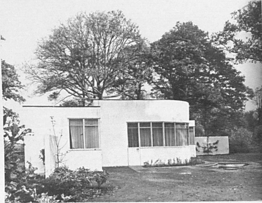
ONE-STOREY HOUSE on a site sheltered by trees on the north and open to fine views on the south. A tank room—often a problem in flat-roofed houses—is fitted in at a convenient break in roof level, where the height of living-room increases. The plan is a development of the basic "Sunspan" plan, exhibited at Olympia in April, 1934.
