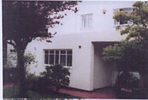
Wells Coates; Sunspan Houses, Wentworth Close, Long Ditton, Surrey.
