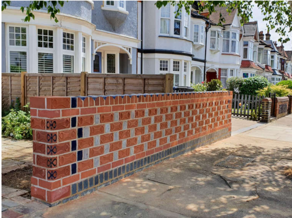
Fig. 4.60. Ornamental wall completed in May 2020 53 (2020)
