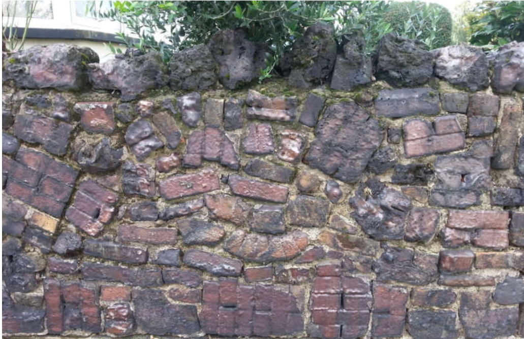
Fig. 4.47. 'Clinker' 48 front garden wall located at the neighbouring house (2019)
