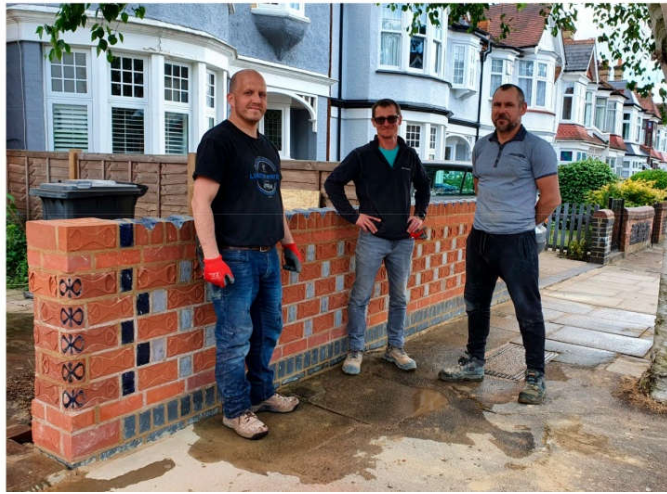
The bricklayers by the completed wall, 24.05.20
