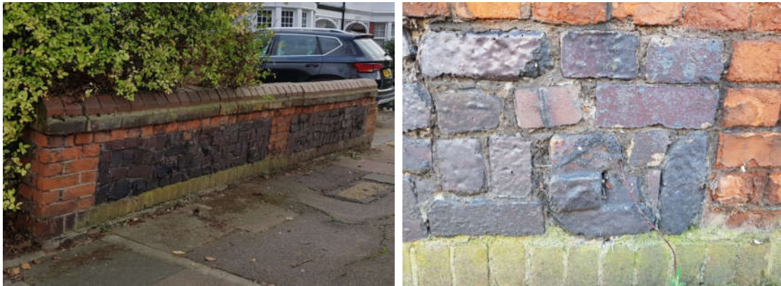
Fig. 4.52. The original wall that was replaced (2019)
