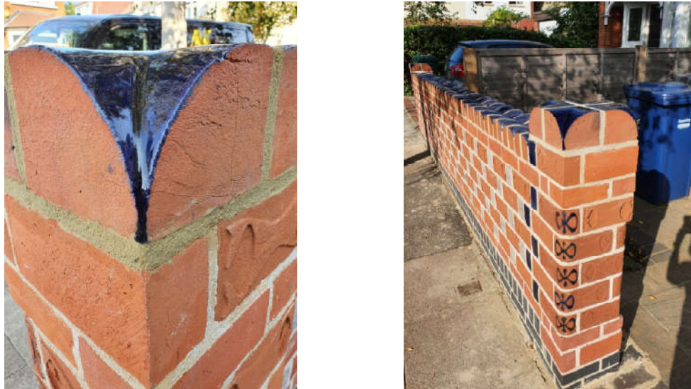
Fig. 4.28. Pier caps for case study 2 glazed by the glaze specialist at the H.G. Matthews factory (2020)
