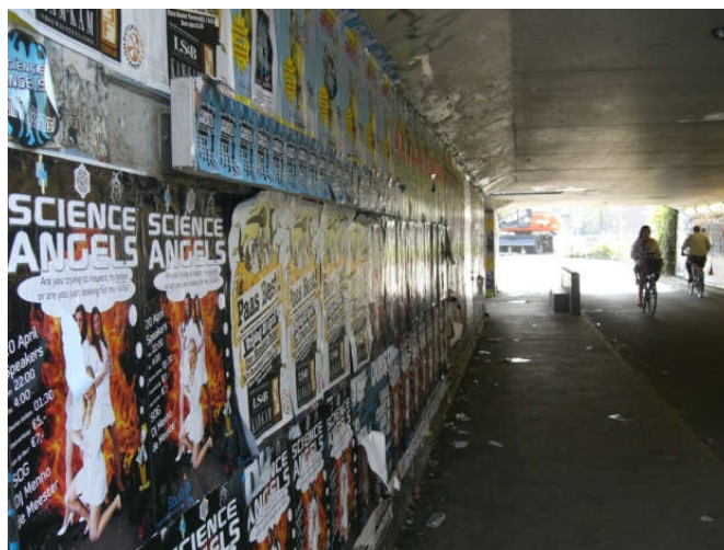
Fig.C.6. Humtunnel, Delft. The tunnel before renovation (Photo: Nagy, 2013)
