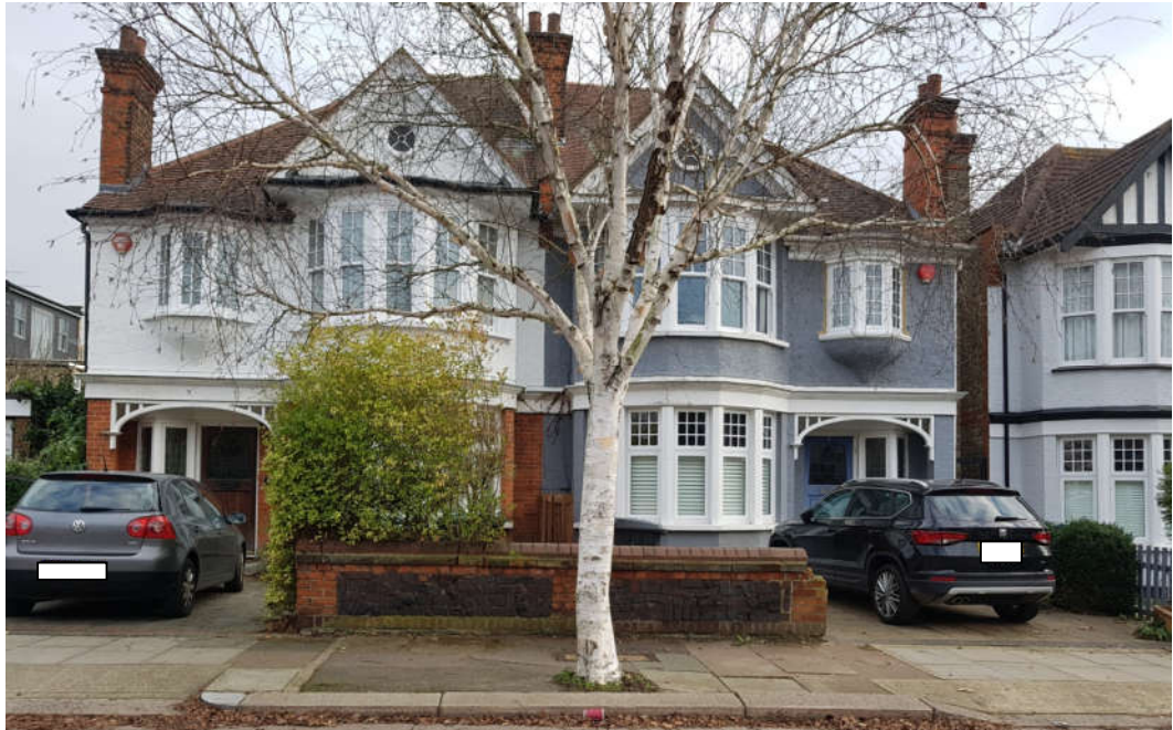
Fig. 4.49. The original front garden wall and houses featuring steep tiled roofs, prominent, jutting gables and timber framing (2019)
