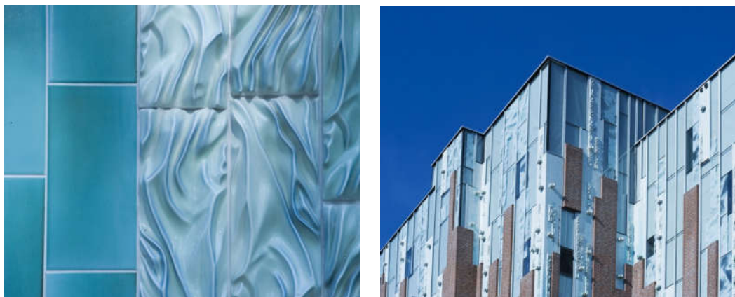
Fig. C.9 Left: elements of porcelain cladding . Right: fragment of the Theatre rear elevation (2021)
