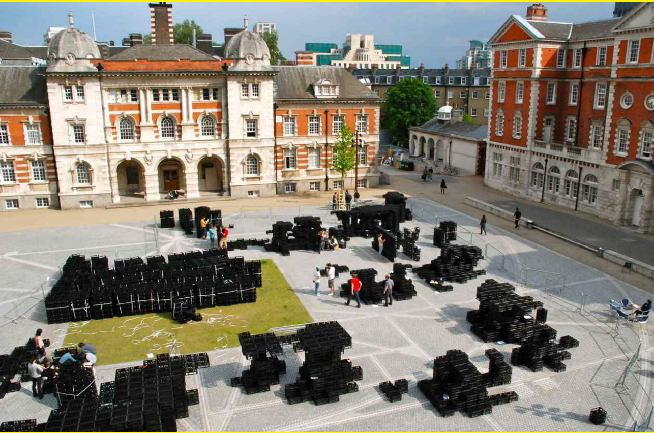
Figure 1.24: PARADE under construction. The bespoke structure was built in public from 4320 black milk crates lashed together with some 30,000 cable ties. This project about being in public was built in public on the Rootstein Hopkins Parade Ground, Chelsea College of Arts (May 2010). Photo credit Marsha Bradfield.
