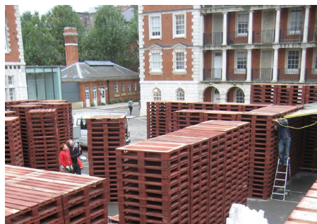
Figure 1.8: Building Atelier Trans Pal (ATP) , an ephemeral structure dedicated to facilitating art/critical and off-site practices. This iteration of ATP took place at Chelsea College of Art and Design (today Chelsea College of Arts) in November and December 2006. It was made of 2000 wooden pallets assembled to make up a space 20m long, 4m high, 7m wide. Photo courtesy of the Critical Practice archives.
