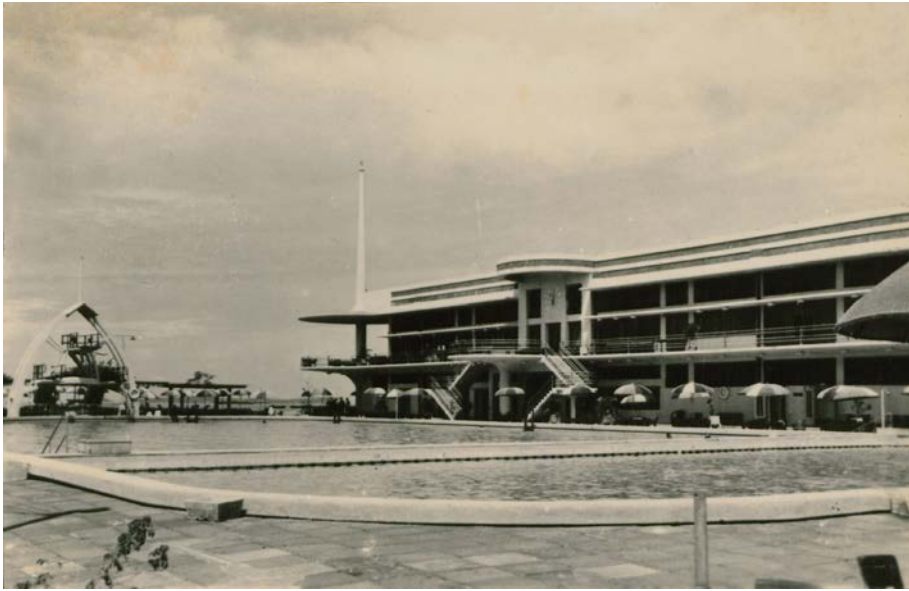
Figure 5. Frank Dowdeswell's 1930s design for the Singapore Swimming Club's new clubhouse, Katong, c. 1950s. Nelson Collection, courtesy of National Archives of Singapore (accession no. 20140000166-0055).
