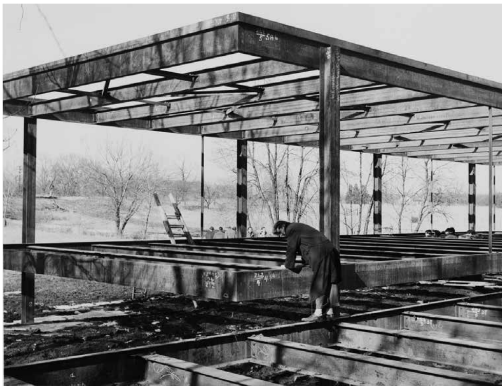
9 Myron Goldsmith, photographer. Farnsworth House (Plano, Illinois) under construction, 1949–50, gelatin silver print, 10.2 x 15.5 cm. ARCH280773, Myron Goldsmith fonds. Canadian Centre for Architecture.
