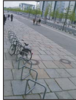
Figure 1.4. Galvanised steel hoop stands, New York
