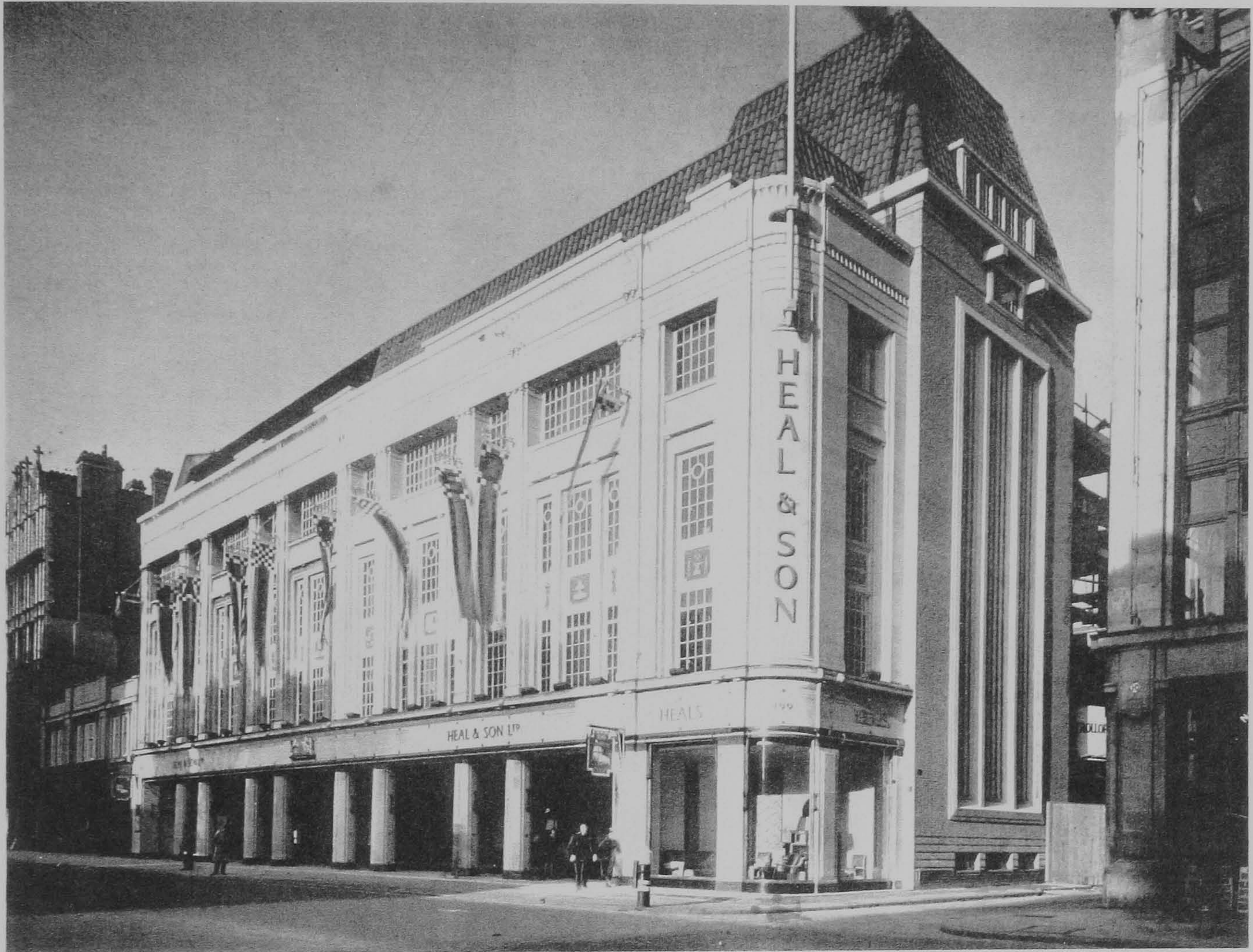
General View. Mr. Maufe carries on the excellent design of Smith and Brewer on the Tottenham Court Road Frontage, but introduces a new character for the frontage to Alfred Mews. The large "Lenserete" window to the new staircase will be noted as well as the extension of the colonnade with its great non-reflecting window.
