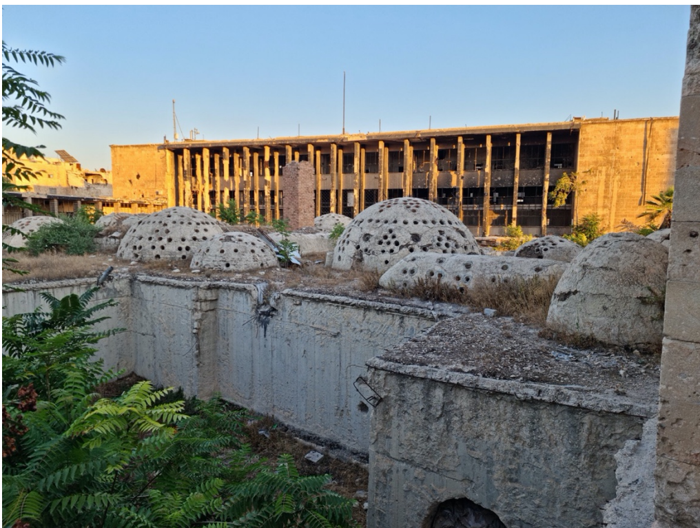
Fig 63. Bottom: Hammam Yalbugha al-Nasir destruction. 2022. Digital photograph: Osaid Hilal.
