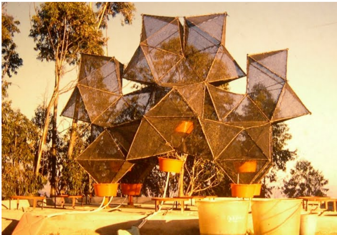
Fig 29. Carlos Espinosa, Macrodiamante fog catcher . 1970. Fog catcher installation (source: integradoatrapanieblas2011.blogspot.com ).
