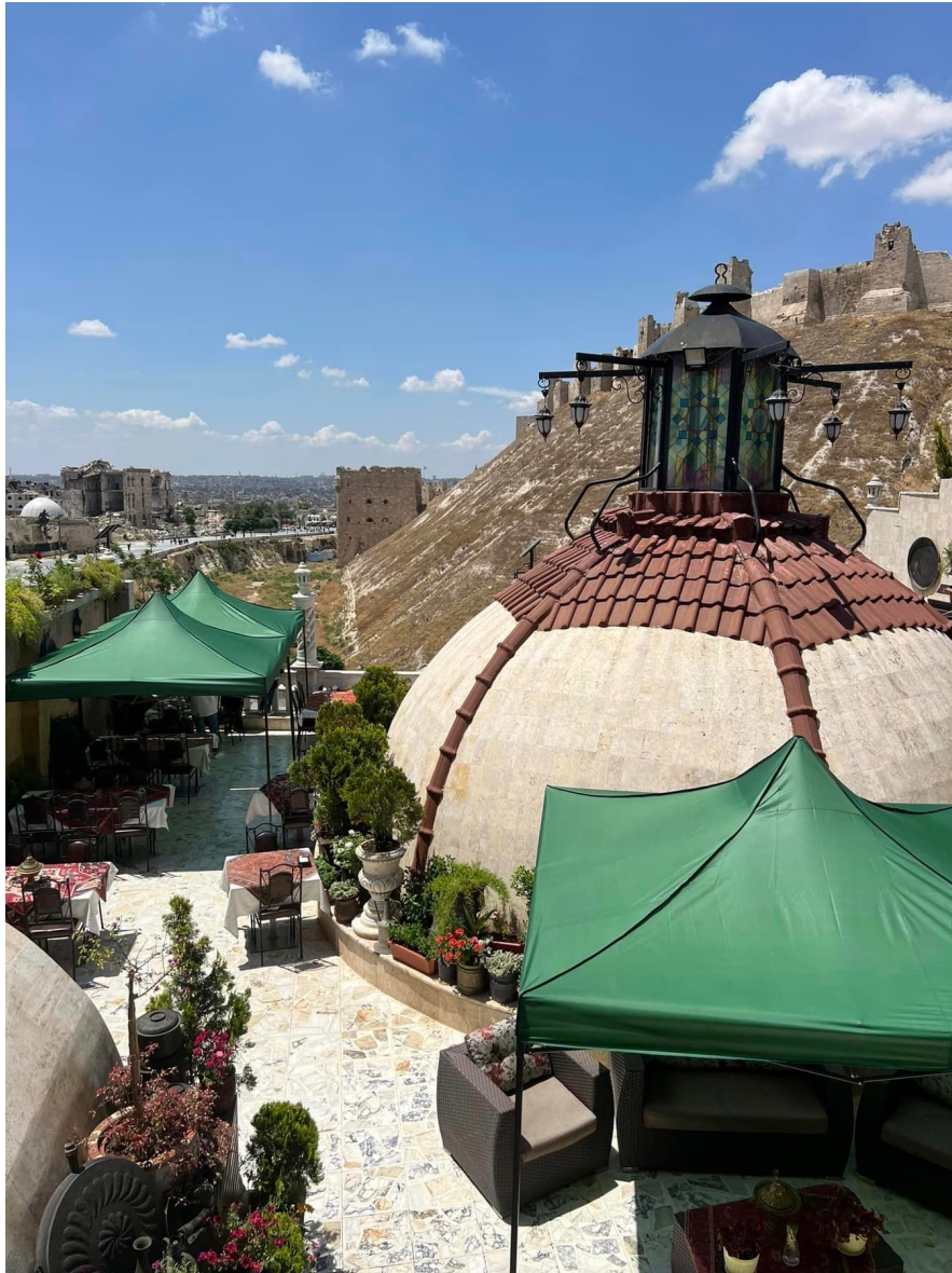
Fig 7. The dome of Hammam Bab al-Ahmar. 2023. Aleppo, Syria (source: The Hammam owner).
