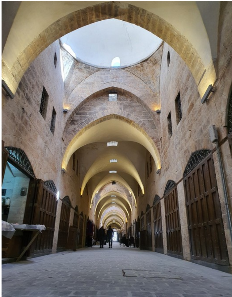
Fig 8. Suq al-Saqatiyya after restoration. 2020. Digital photograph (source: thebestinheritage.com ).
