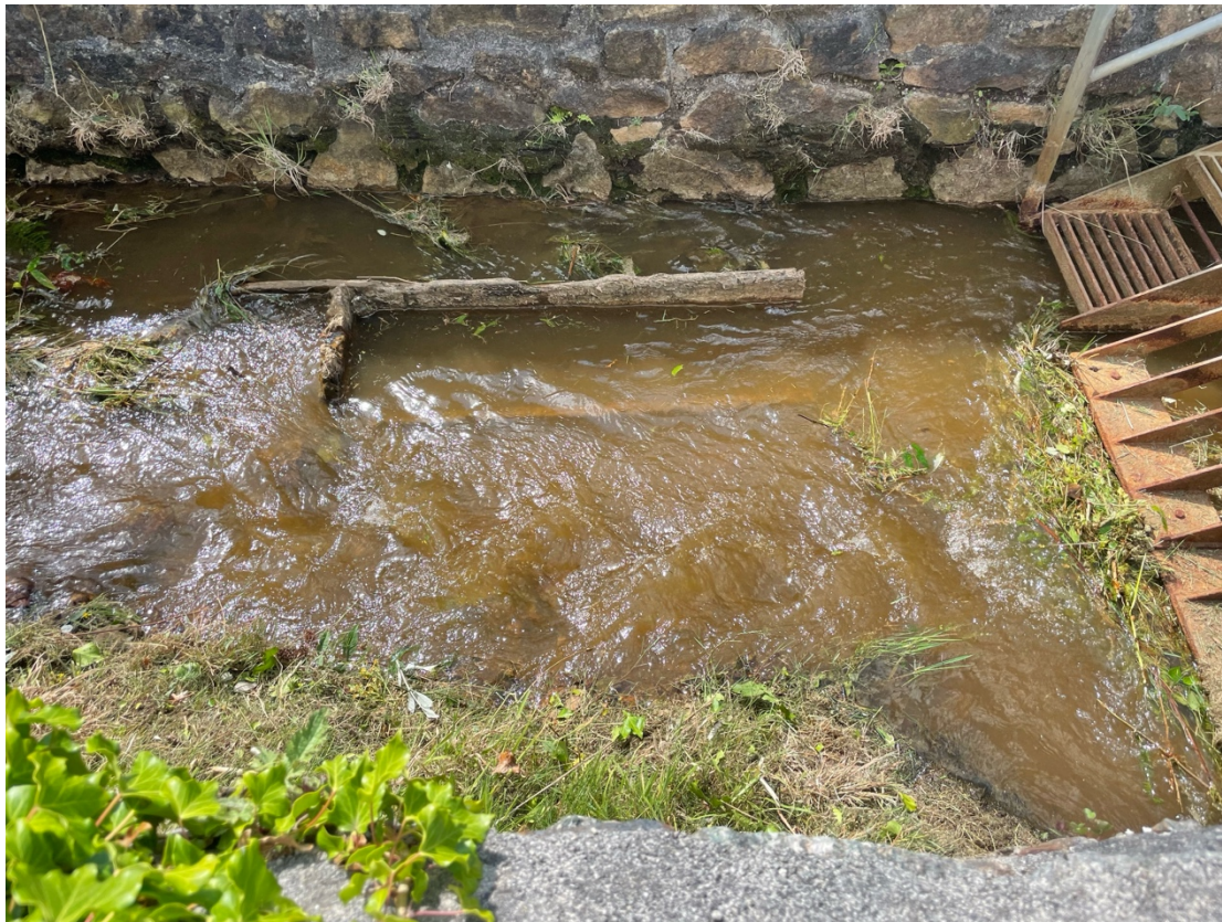
Figure 3.8 Contextual image: Chapel Road, near the bridge. Photograph by the author, 2022.
