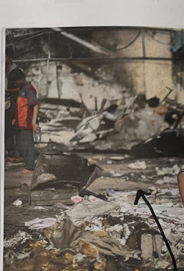
Fire engulfed everything'
