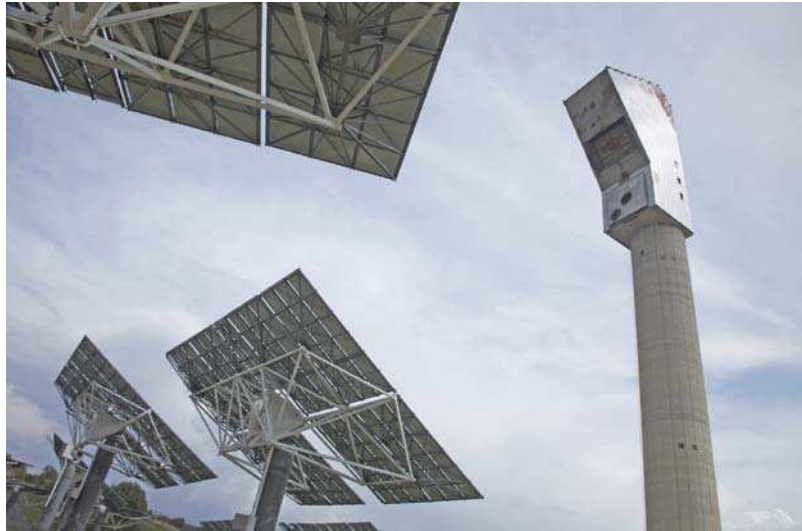
Fig 11. Heliostats facing the collector tower. Thémis centre, Targassone, France, 2010.
