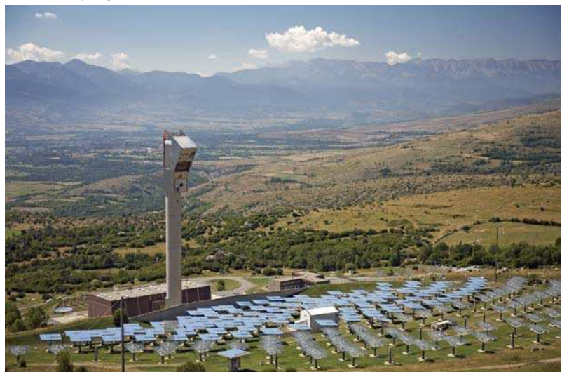
Fig 9. Thémis solar power station. Targassone, France, 2010.
