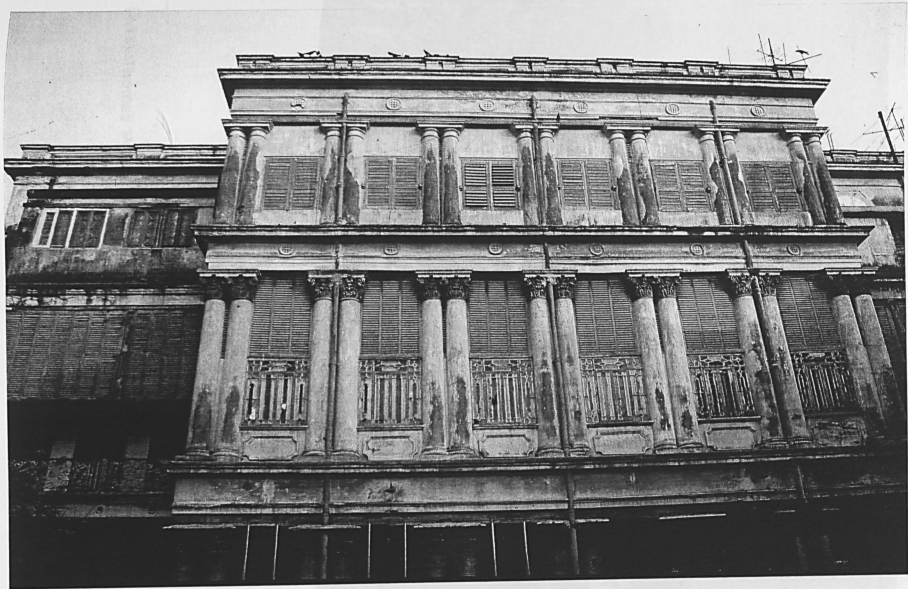
(2.12) Building opposite Marble Palace, with misplaced classical orders
