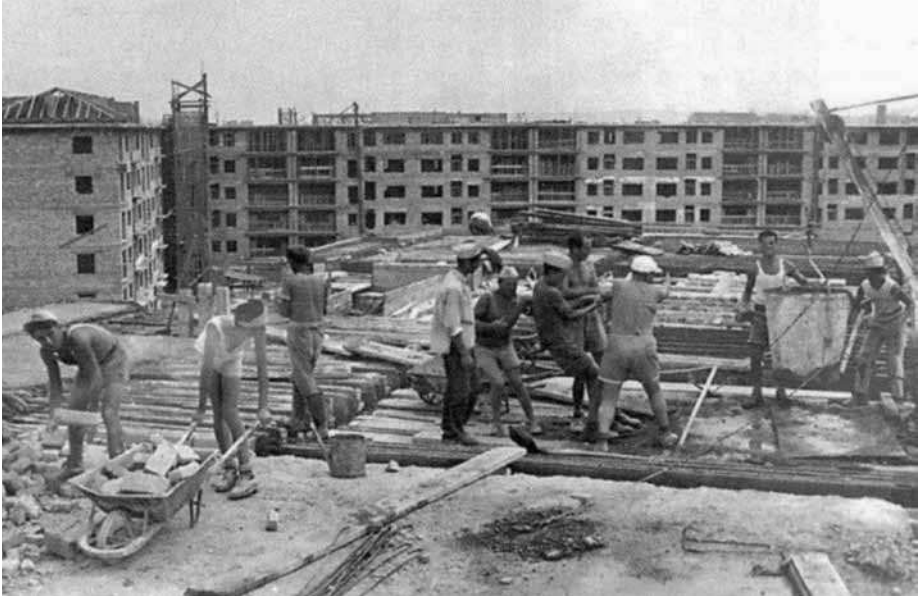
Figure 2: Workers in New Belgrade, pavilion 14/15. Source: Stare Slike Novog Beograda Facebook group, https://www.facebook.com/pages/Stare-slike-Novog-Beograda . Used with permission.
